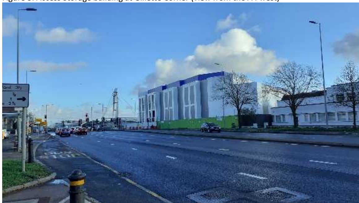
Figure 3. Access Storage building at Gillette Corner (view from the A4 west)
