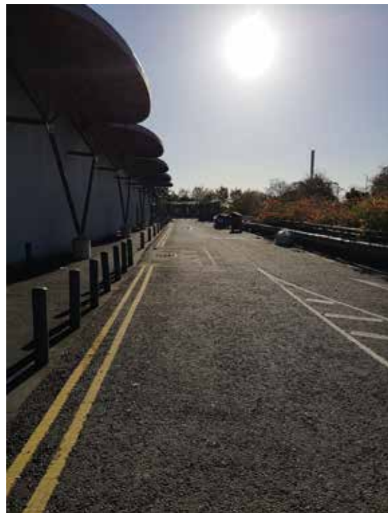
Access Road to the Delivery Yard
