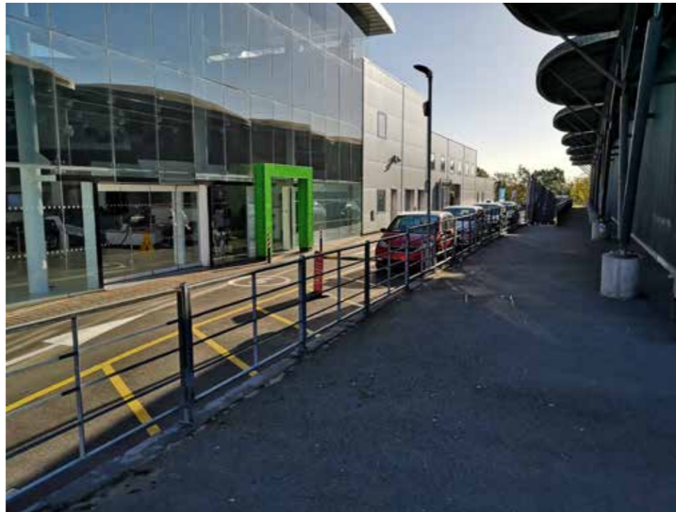
Site Boundary along the East
