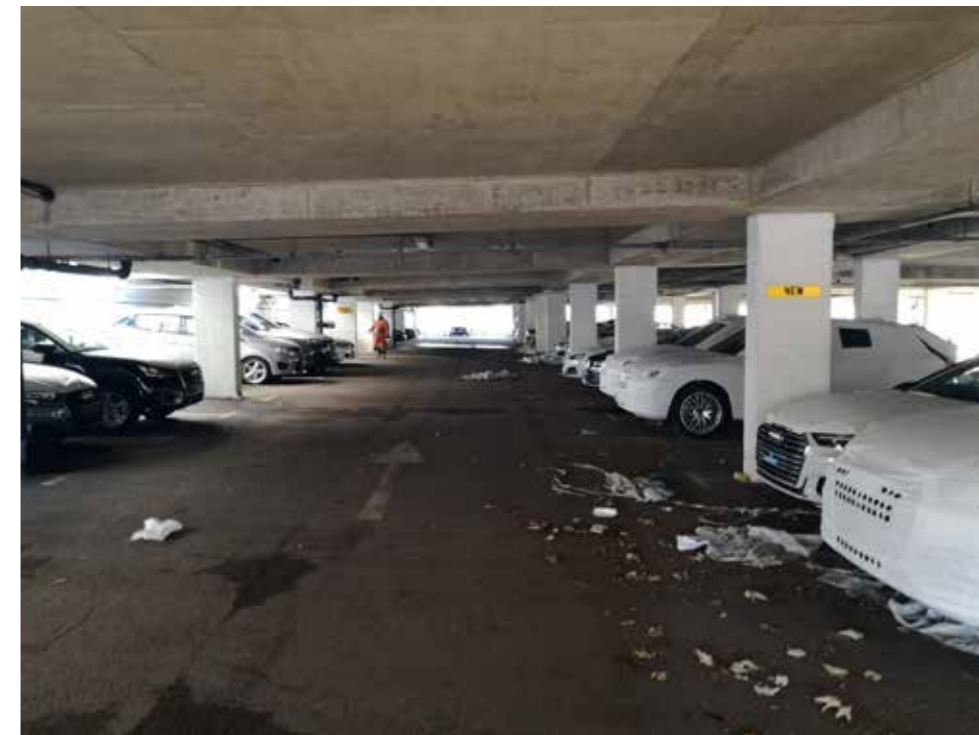
Undercroft Car Park
