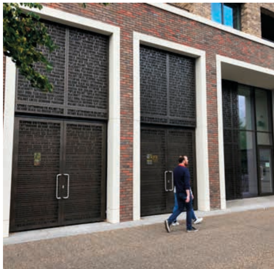
Decorated metalwork panels and doors screening sub station/ancillary uses
