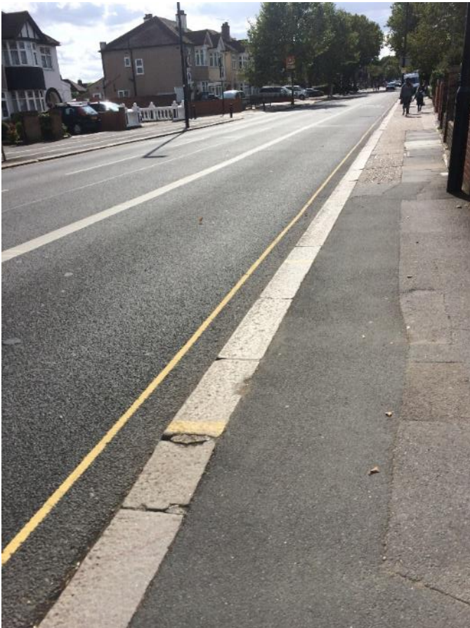
Insert 5.5: Route 4 - Photo Location 4
