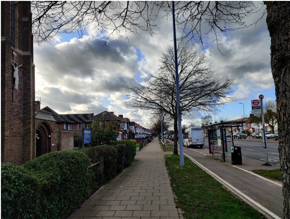
Insert 7.6: Route 7 - Photo Location 5
