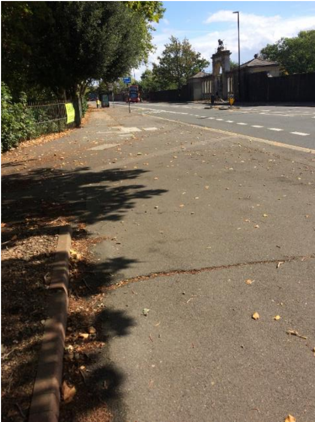
Insert 4.6: Route 3 - Photo Location 5
