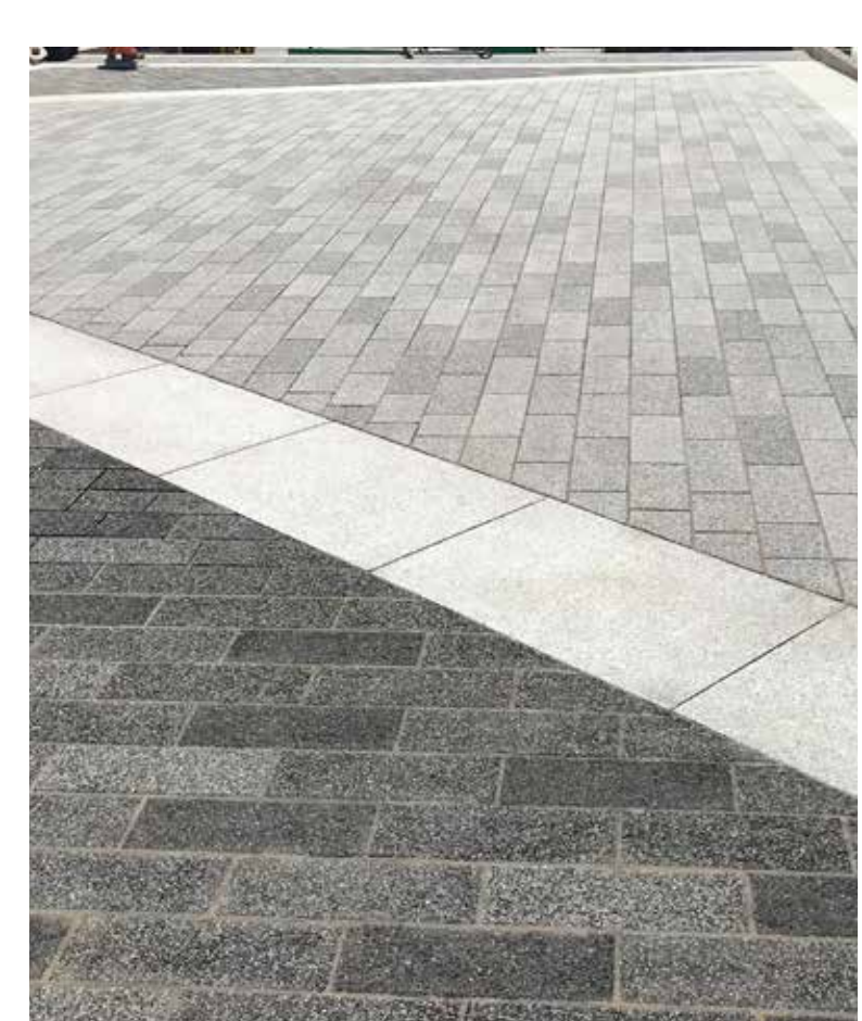
Continuous high quality paving finish incorporating robust mixed tone block paving and stone banding
