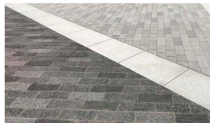
Continuous high quality paving finish incorporating robust mixed tone block paving and stone banding
