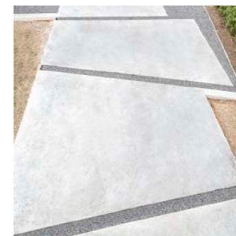
Feature paving to core entrances
