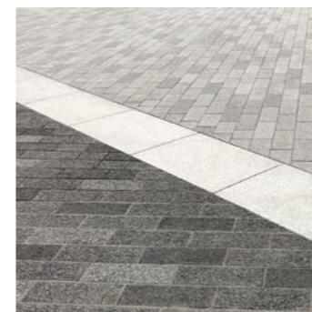
Dark-grey and light-grey block paving with natural stone banding
