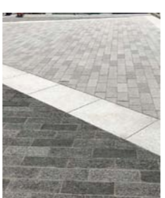
Continuous high quality paving finish incorporating robust mixed tone block paving and stone banding
