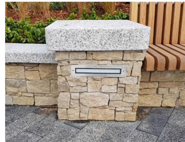
Recessed linear lighting
